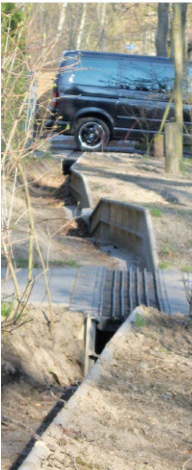
Compensating for height differences
