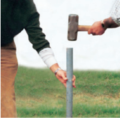
Positioning the posts
