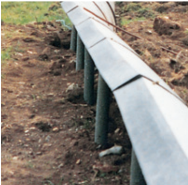
Assembling the fence panel with final topsoil backfill
