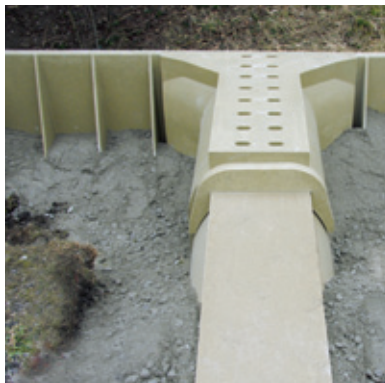
Building the entrance area with near surface tunnel
